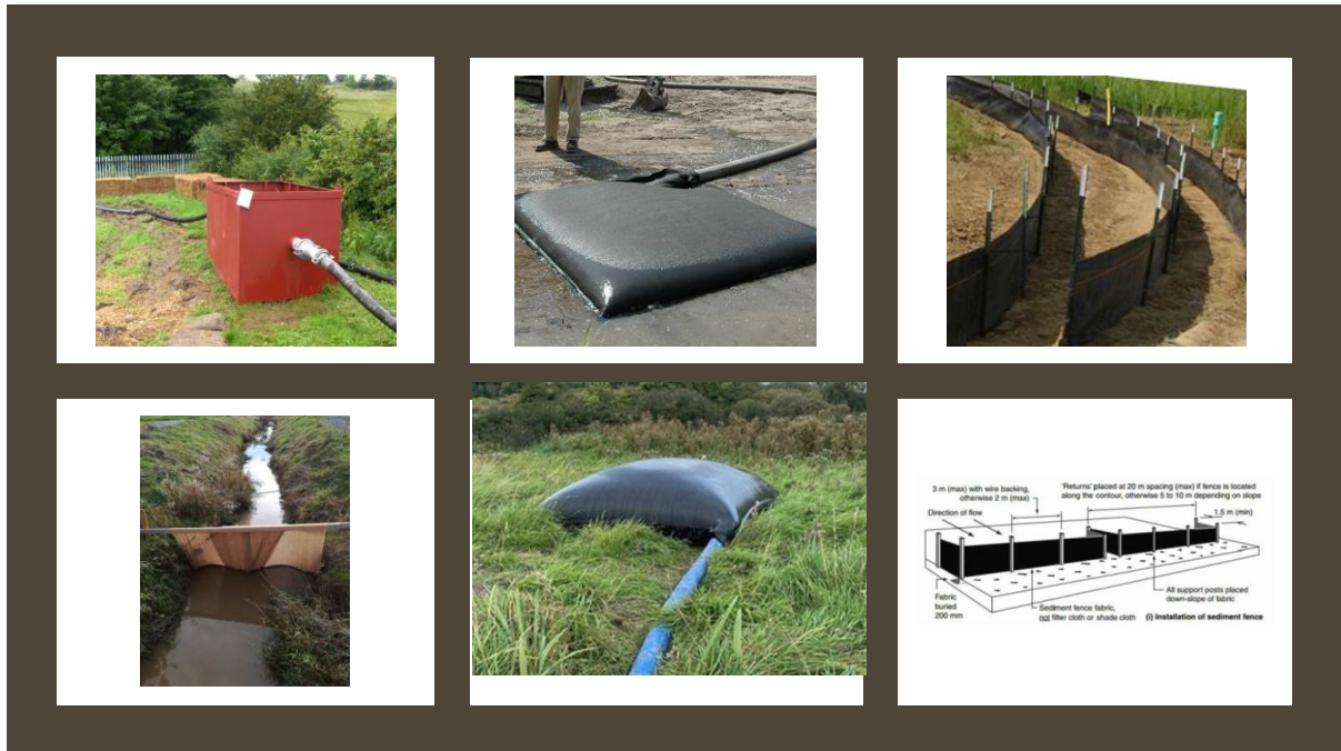
Figure 2-9: Examples of Proprietary Silt Control measures
