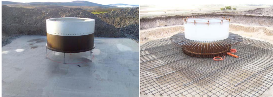
Plate 2-2: Levelled turbine tower “can” Plate 2-3: Steel reinforcement being added
